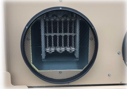
10KW Resistance Heater Kit
